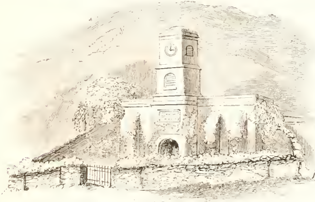
TANK AT NORTH MALVERN.
